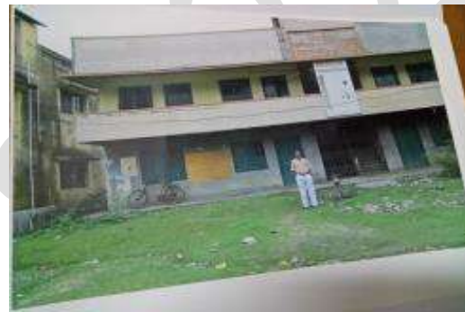
Kandapasara Flood Shelter
