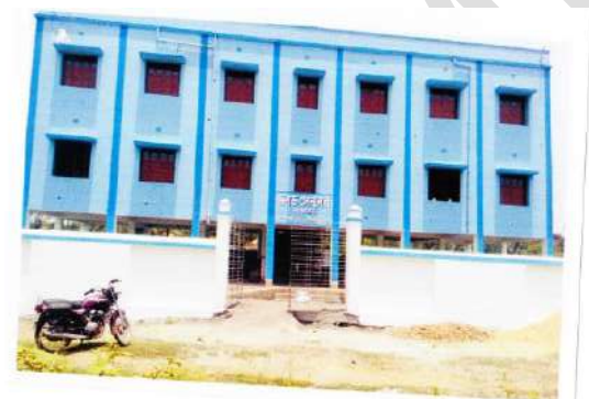
Naranda Flood Shelter
