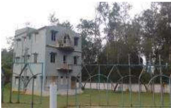
Dakshin Balarampur Flood Shelter
